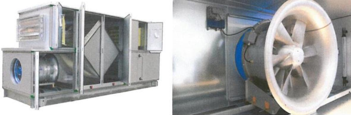
ill.1: Usage of a high performance axial ventilator (detailed right).
